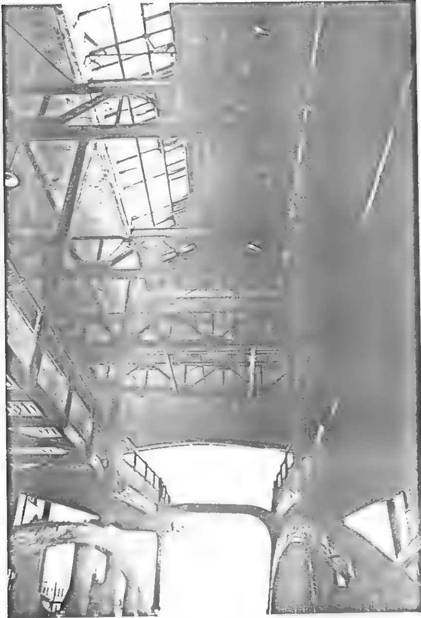
Ferryslip C slylight.
